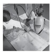
(3) Rewet the felt if the specified liquid dishwashing detergent solution has not completely penetrated, if drying occurs, or if dry felt is exposed during scraping. Pick up the scrapings while still wet as they are removed from the floor and place in a heavy-duty impermeable trash bag or leak-tight container. Wet-scrape all felt from this floor area before proceeding further.
