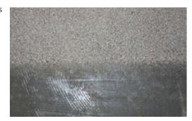
**CSP1 Profile** Top CSP-1 | Bottom before grind
