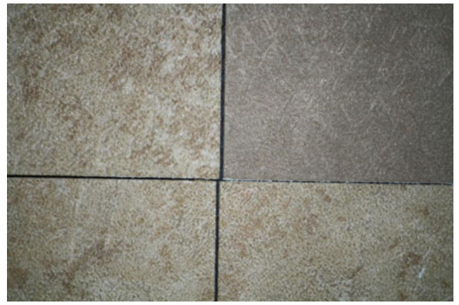
Photo 10: Result of severe underfloor humps.
