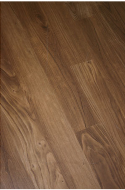
Photo 9: LVT installation meets ASTM-710 Standard for flat subfloor.
